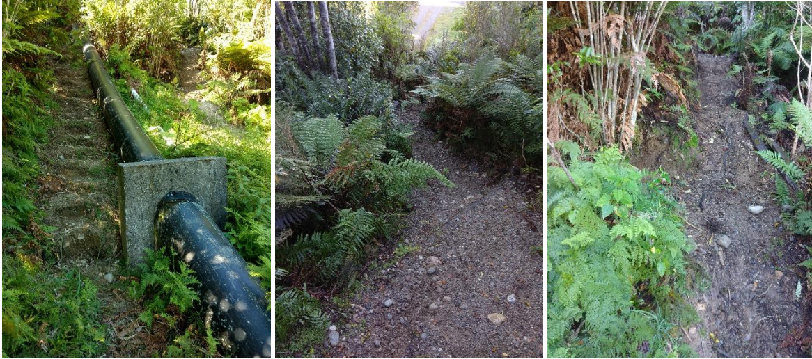
Current situation showing pipeline and rough track
